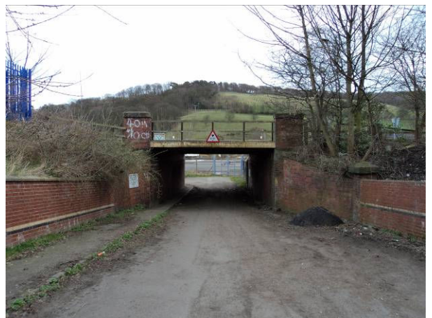
Image 3.8: Height restricted railway bridge
