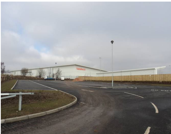
Parking to the eastern boundary
